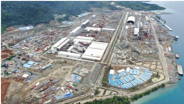
Photo of the PT ZhongTsing New Energy Project
